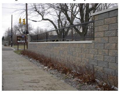
revitalization plan under taken by the town. Other systems utilizing piers were eliminated due to existing fiber optics running the length of the wall resulting in the selection of Concorde to set the precedent. A Concorde wall of the same design was recently completed in the neighboring community of Moraine to continue the unified appearance the length of Dixie Highway entering both communities.
